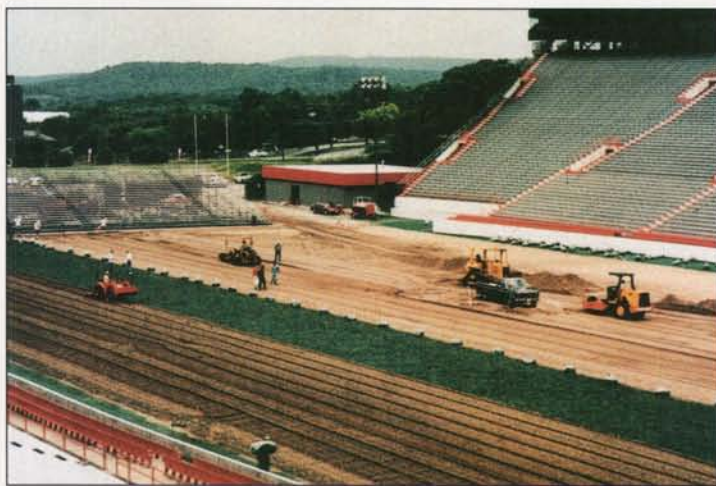
A layer of crushed gravel was laid as a sub-base and topped with 10 to 12 inches of a sand and peat mix.
