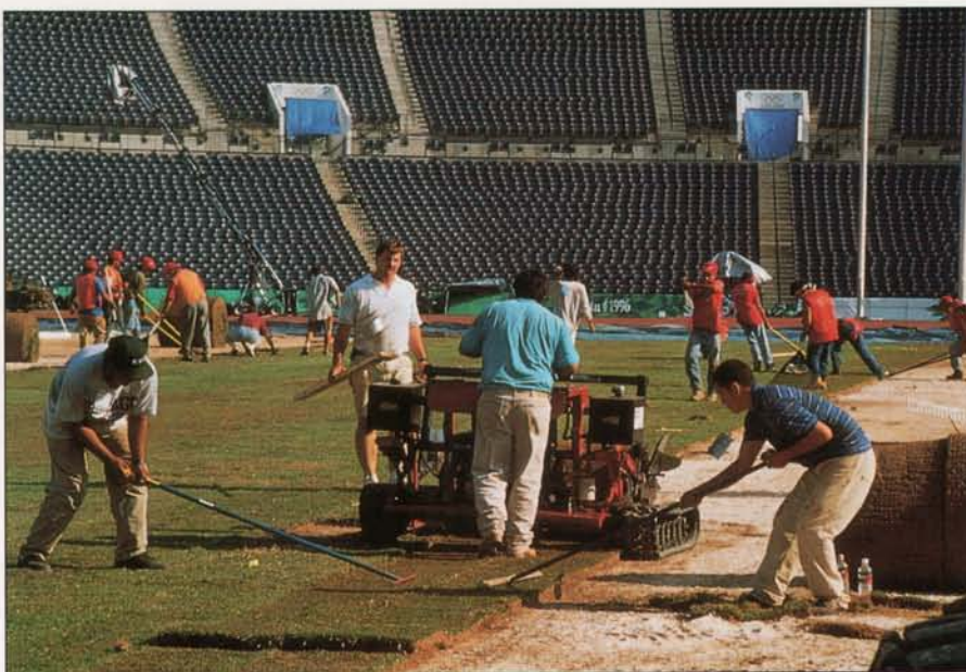
Racing the clock, crew members push and pull strips of sod into place. Photo courtesy: Steve Hogben, Valley Crest Inc.
