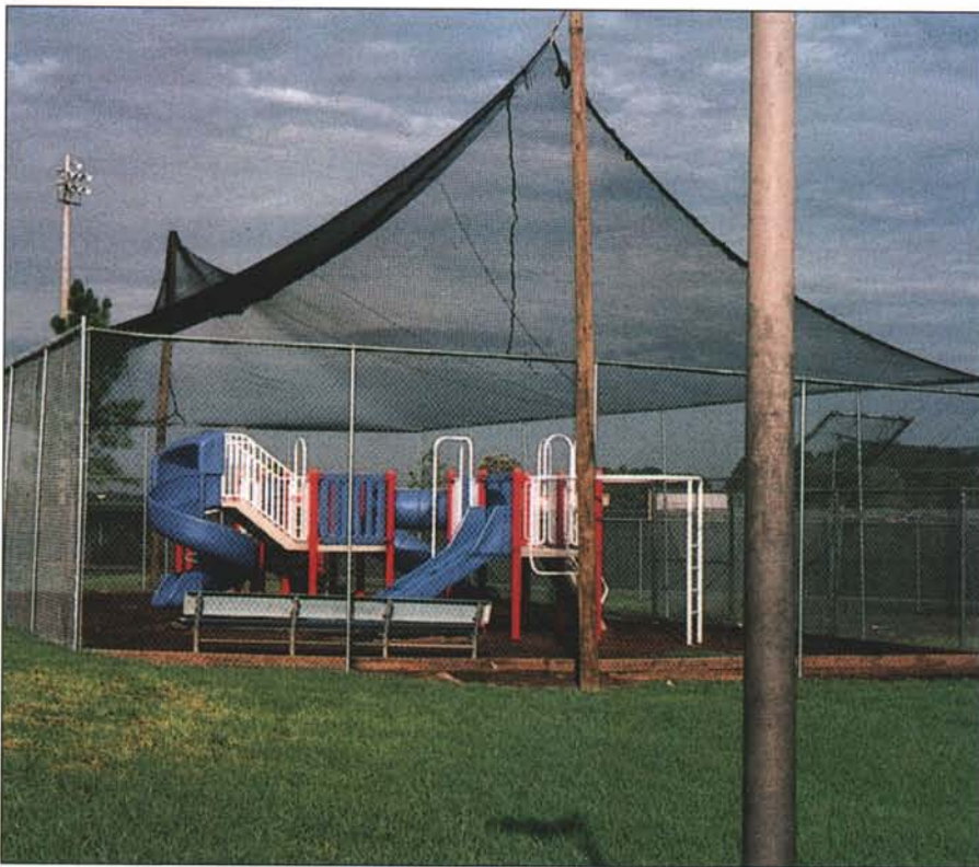
Evaluate all aspects of your facility to decide where priorities should be placed. In some parks, for instance, it might be reasonable and prudent to fully enclose a "tot lot."
