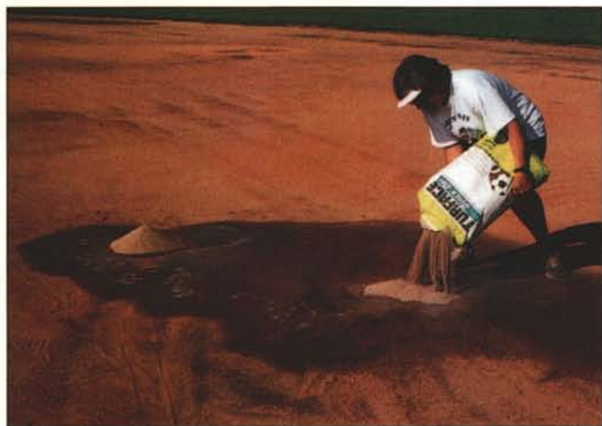
Calcined clay (and other drying agents) can soak up puddles that are less than two inches deep.
