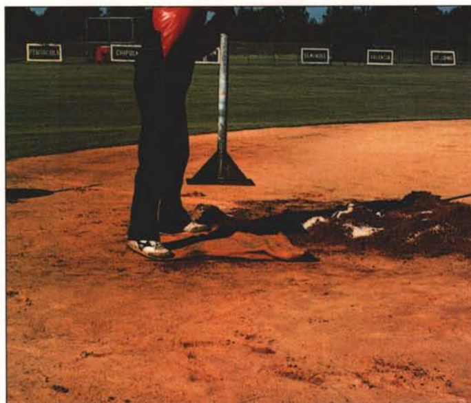
French Drain — Step Four. Tamp approximately two inches of loose clay over the opening for consistent and even playing surfaces.
