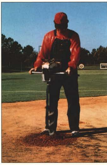
French Drain — Step One. Use a fence-post auger (which can be rented) and dig multiple holes into the heavily compacted soil. For larger areas, a telephone-pole auger can be used.
