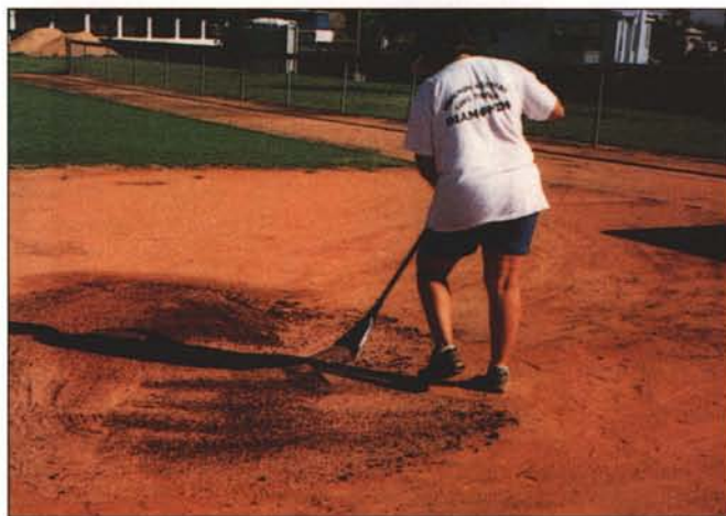
After calcined clay has been raked smooth, a field should be ready within about 20 minutes.
