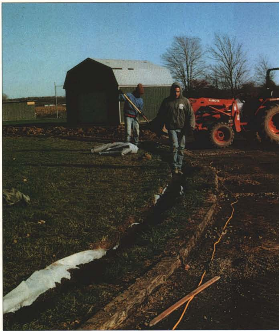
Installing a "sand drain" along the inside of a track can help to drain both the track and the field area inside.
