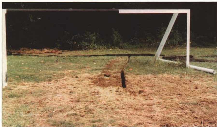
Strip drains can be used to target problem areas, like this one in front of a soccer goal.
