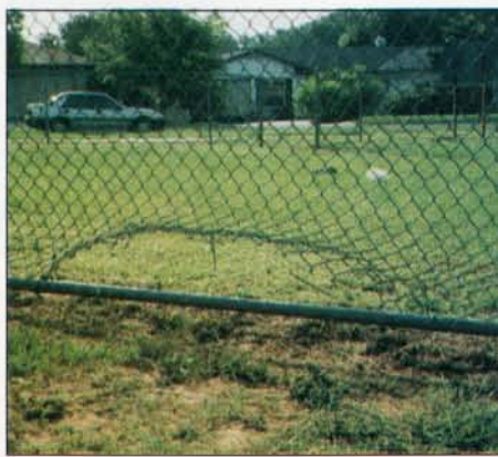
Improperly constructed, damaged or loose fencing creates a potential for injury to both players and spectators.
