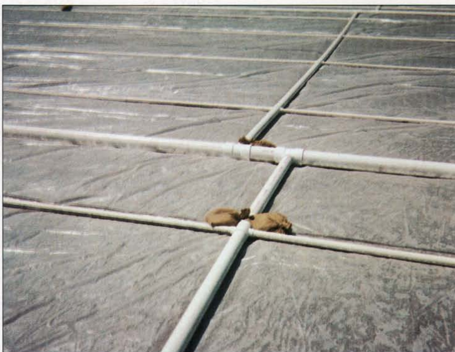
The field's new drain lines, a vast improvement over the previous system, are made of Schedule 40 PVC pipe with solvent weld joints. This technique forms a rigid monolithic drainage system that can pull 80,000 gallons of water per hour off the field.
