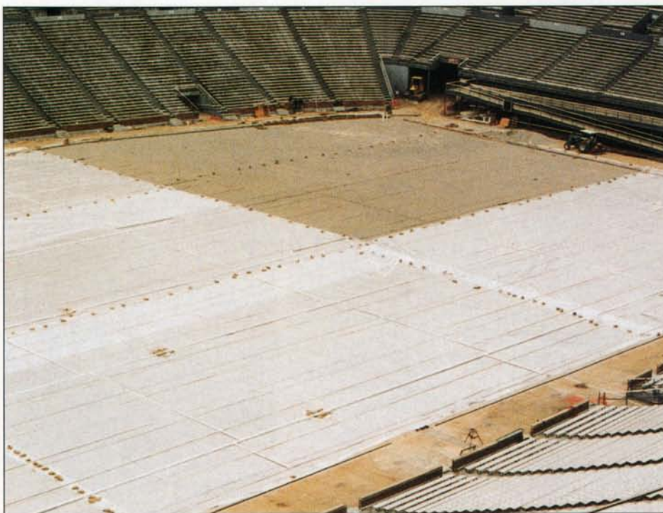
The irrigation system and drain lines were covered by 8,000 tons of sand to provide a good base and optimal drainage.
