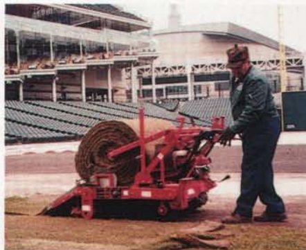
INSTALLED CLEVELAND INDIANS IN 42" AND 48" ROLLS
