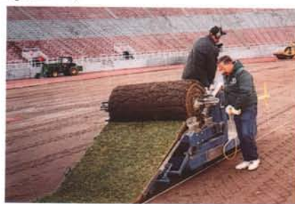
INSTALLED OHIO STATE (AND STRIPPED) 2" THICK TURF 48" ROLLS
