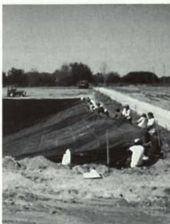
STORMWATER RETENTION POND
