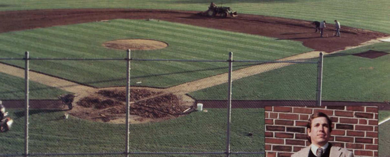
Twi-Light Field. Infield skinned-area construction.
