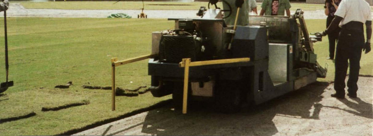
A Cynet 48 turf-installation machine was used to install the baseball field for the Florida Marlins at Joe Robbie Stadium. Photo courtesy: Cynet Turf.
