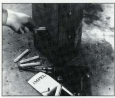
IMPEL Rods are molded from waterdiffusible boron, a natural element recognized as an effective deterrent to rot. The resemble glass rods and are inserted into small holes drilled in wood where it is most susceptible to rot.
