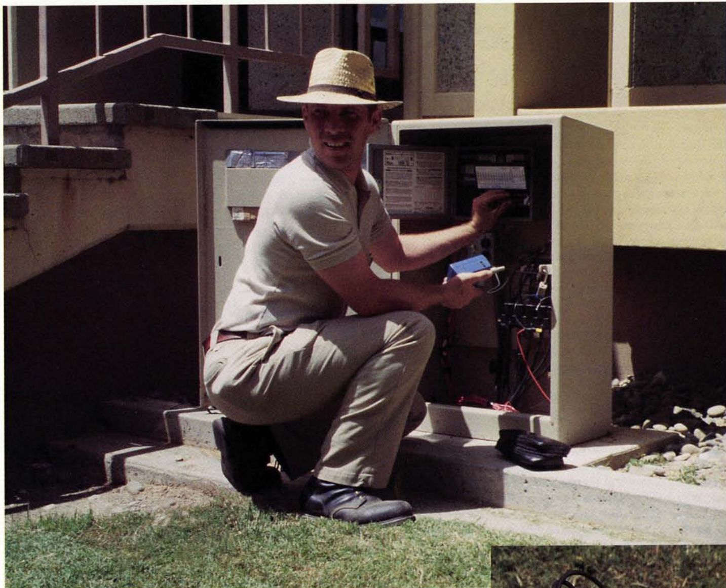
Mark Satterfield, UC Davis irrigation technician, trouble-shoots a wiring problem with an irrigation control wire analyzer. Photos courtesy: Bob Milano. (Inset) Close-up of an irrigation control wire analyzer.
