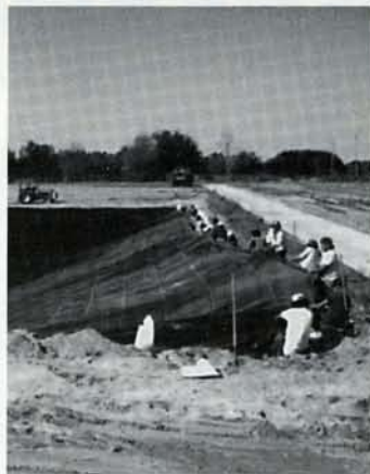
STORMWATER RETENTION POND
