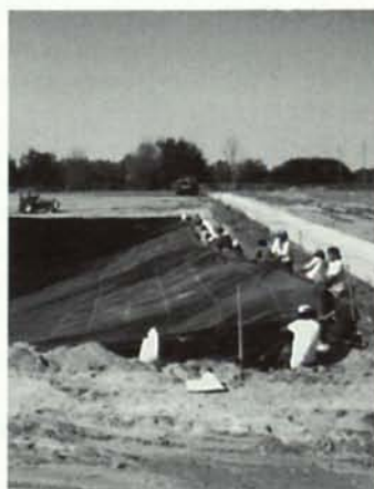
STORMWATER RETENTION POND
