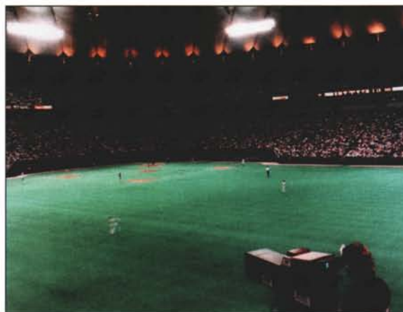
Indoor lighting for the Metrodome in Minneapolis, MN. Light levels of 200 to 300 footcandles are necessary for good color rendition of television transmission.
