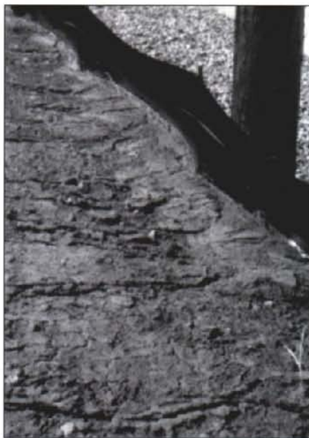
Silt fence installed to capture sediment. Photo courtesy: Jerry Fifield.
