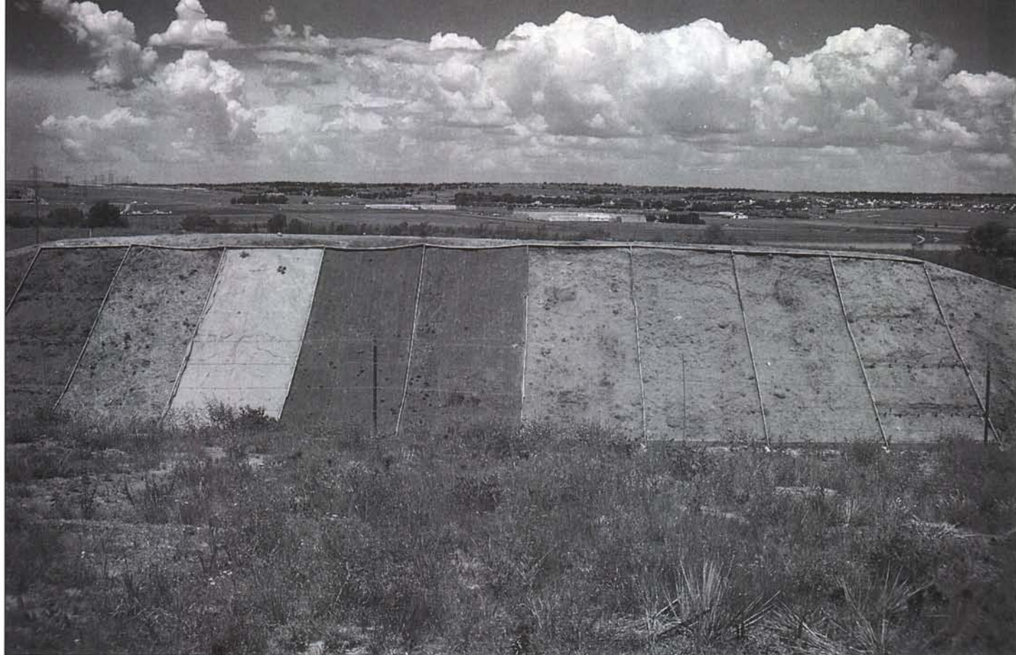
Erosion control products on test slope (L to R): wattles, wood fiber hydraulic mulch, paper hydraulic mulch, bare ground, jute, coconut fiber mat, polyester blanket, and hay with tackifier. Photo courtesy: Hydro Dynamics.
