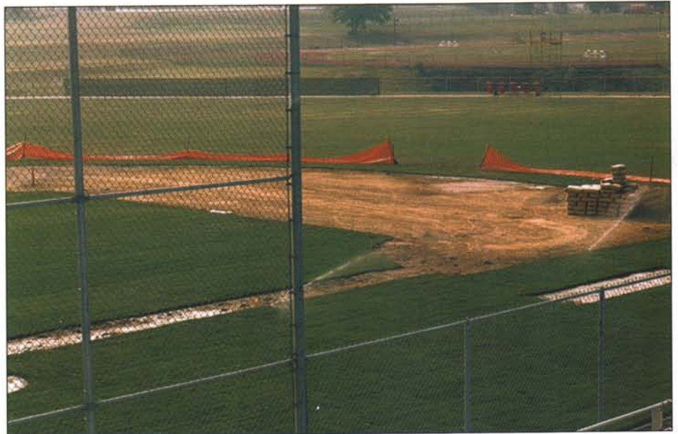
Redbird Field infield under construction.
