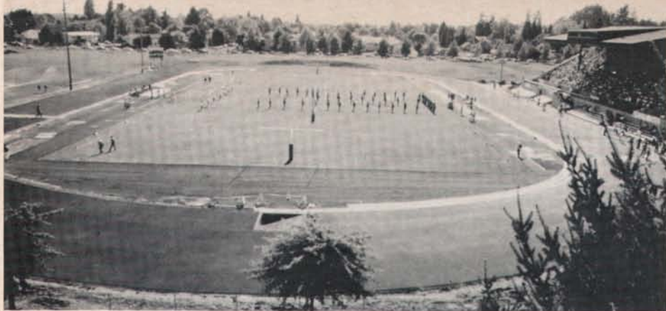
Stadium field and track following renovation.
