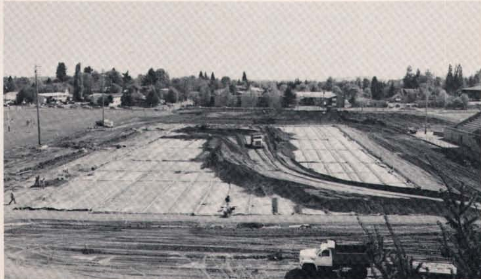
Sand is carefully laid over drainage/subirrigation network.
