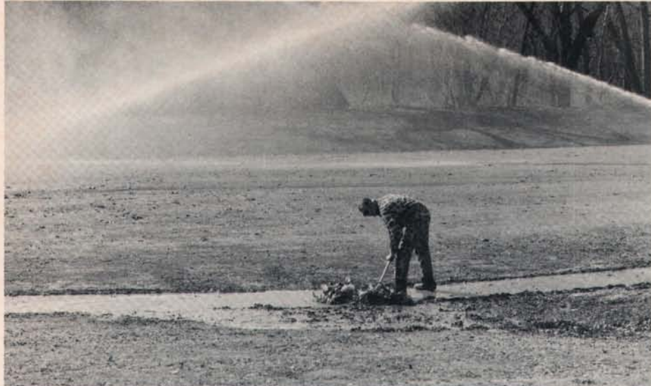
Crew member uses squeegee to push silt into new storm drains following a recent flood.
