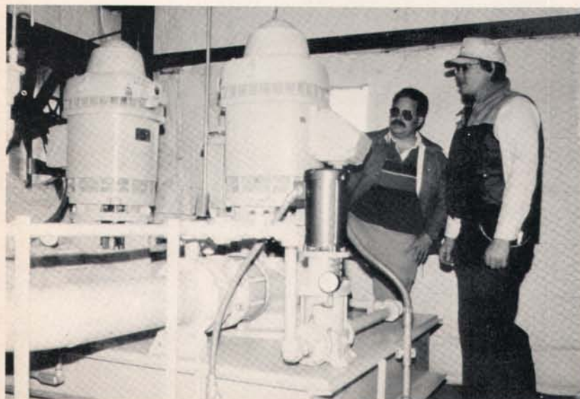
Murray (left) and Hartline (right) check new pump station.
