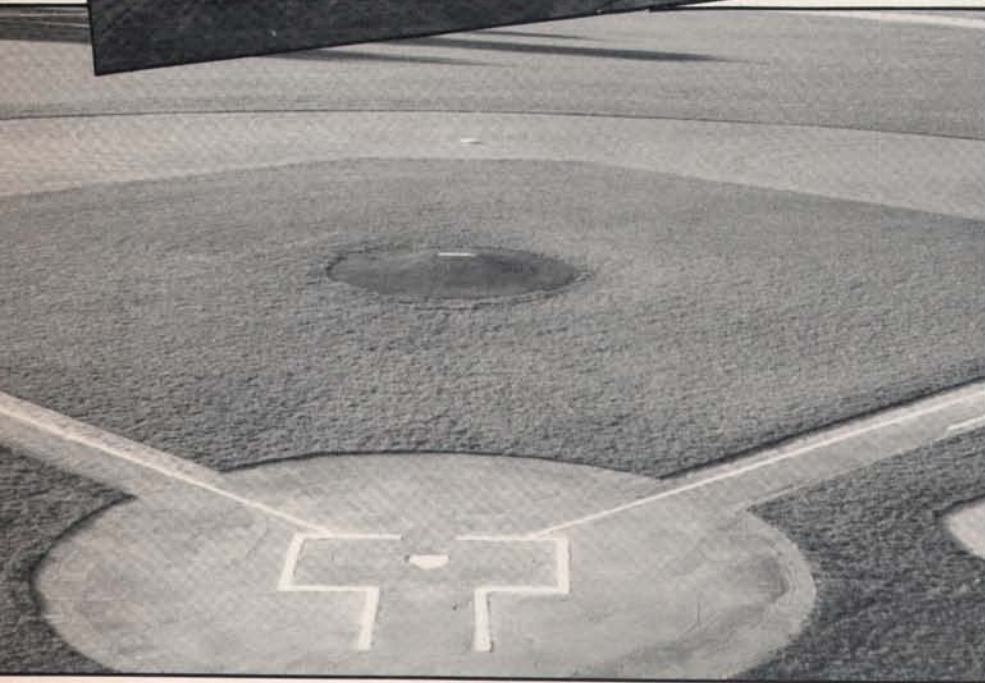
Removing built-up infield dirt with Grade-all (top). Finished diamond marked and ready for a game.
