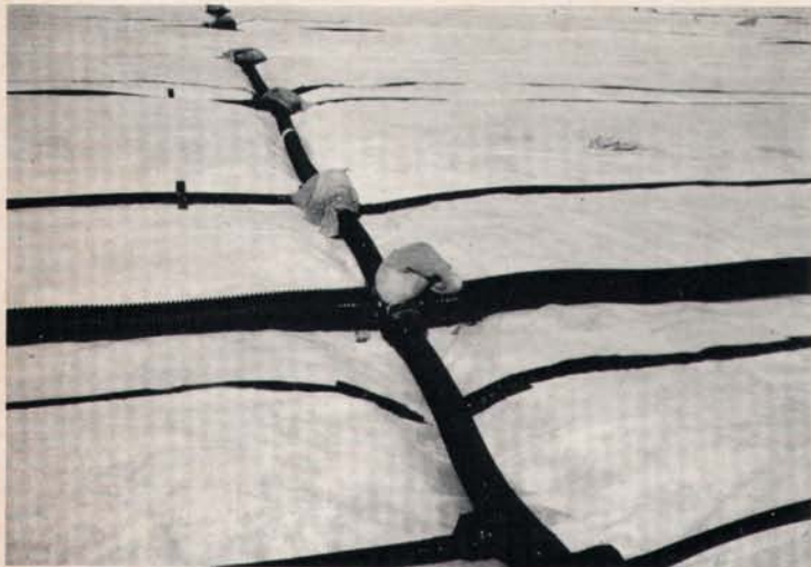
A network of drainpipe on top of a moisture barrier serves to drain and subirrigate the PAT system.
