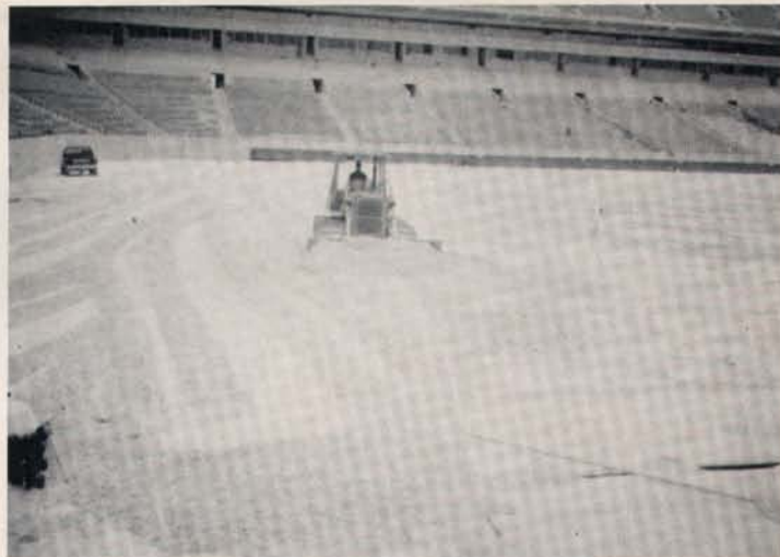
A foot of sand was carefully spread over the drainpipe.
