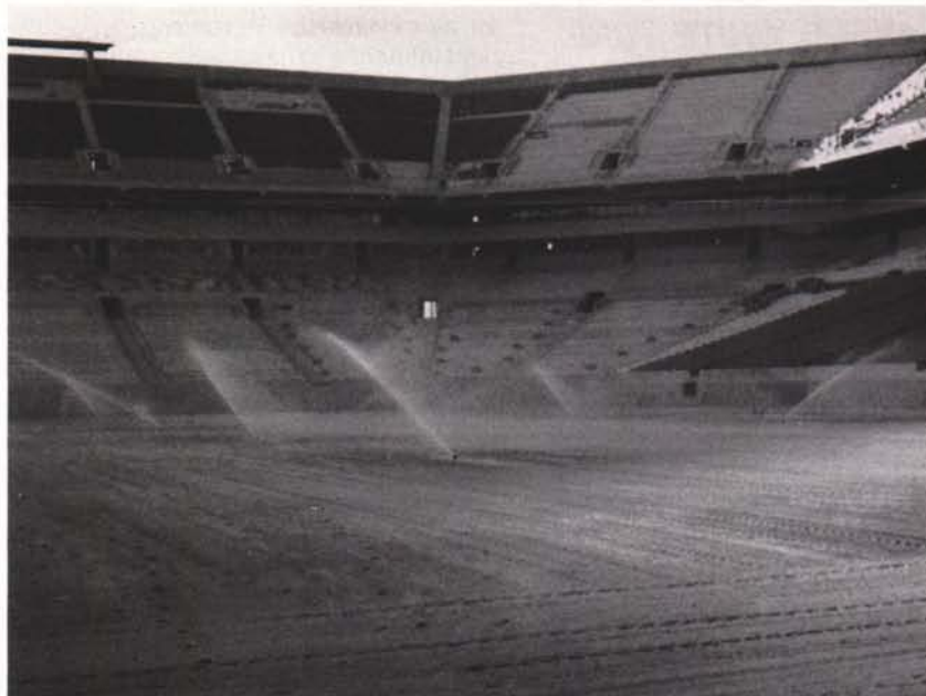
After calcined clay was mixed into the top three inches of sand, the field was irrigated to bring moisture levels up to specifications.
