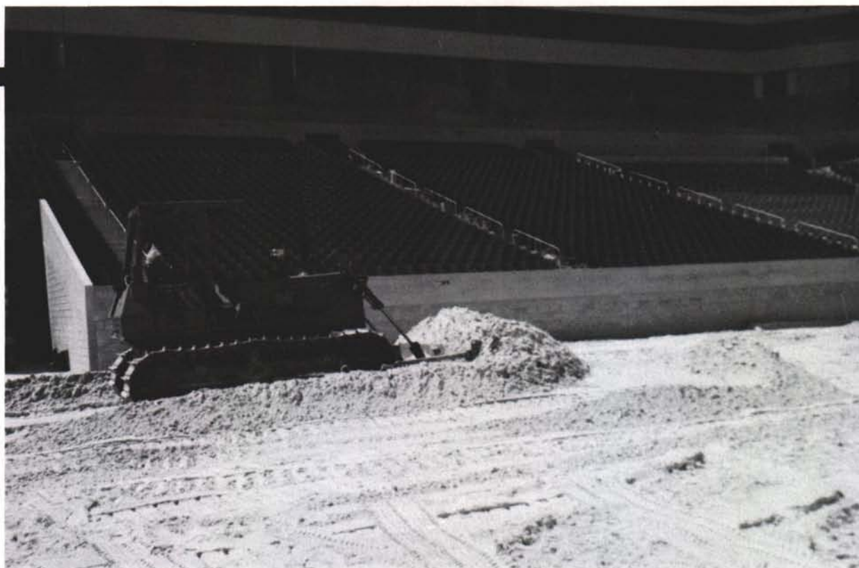
More than 8,000 yards of sand were graded to a four-inch crown.
