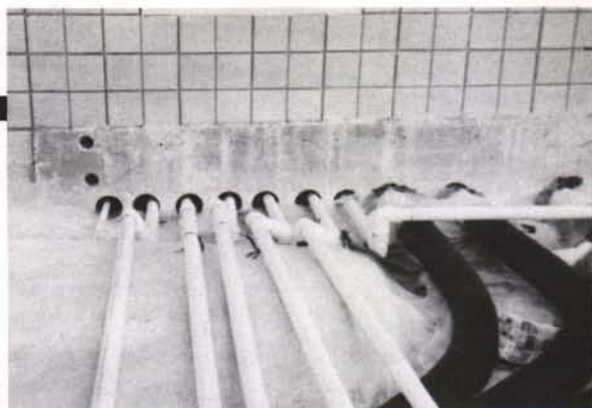
Irrigation and drainage lines lead into a central control room.
