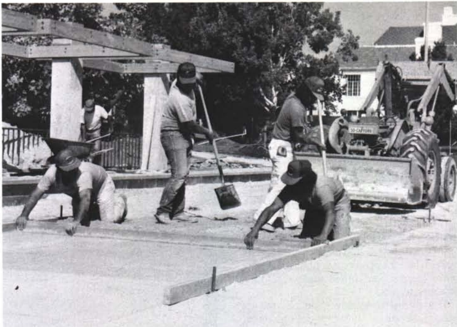
To come within a 1/16 inch tolerance on the greens at Roxbury Park, the crew from American Landscape Inc. installed the sand like they would concrete.
