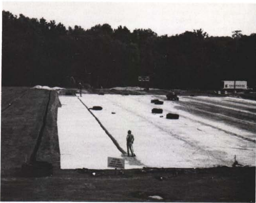
The subgrade of both artificial fields was covered with geotextile fabric before perforated drain tubing and sand were installed.
