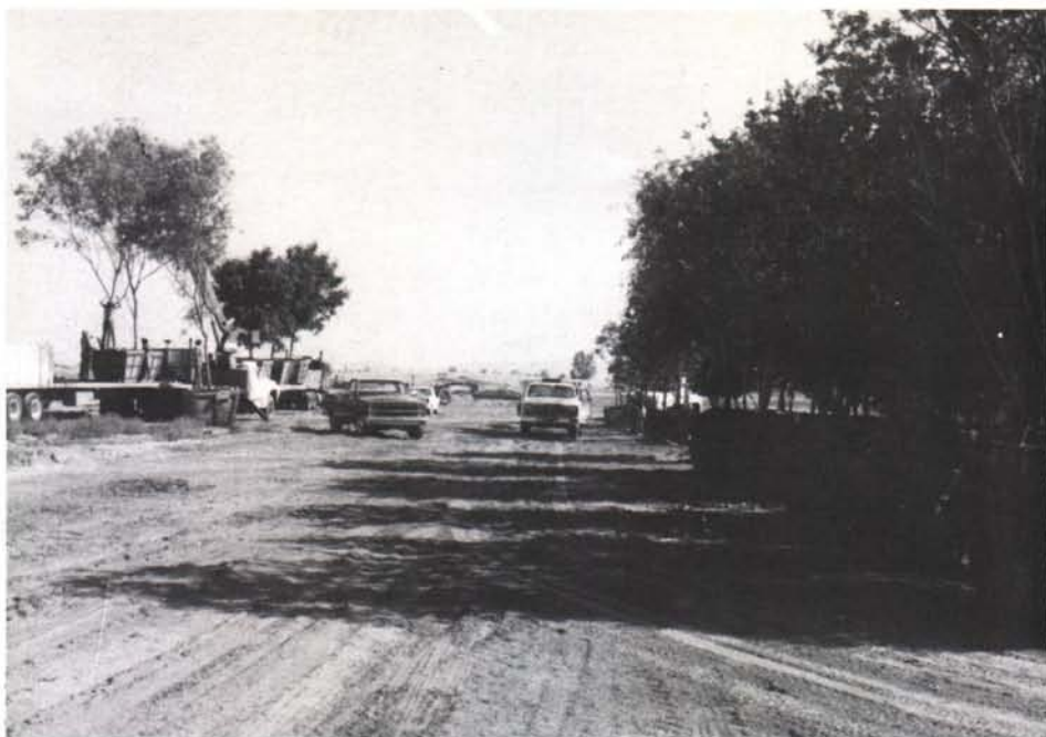
More than 1,500 trees were planted on the Arroyo nine. This proved to be one of the more difficult tasks of the entire project because of extremely hot weather.
