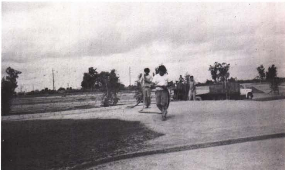
In several areas of the course, hydroseeding was performed for erosion control purposes.
