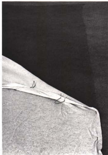
Wire loops hold the fabric down and can be installed quickly.
