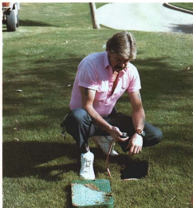
Richards Jenkins, irrigation supervisor at Gainey Ranch, checks the valve output pressure to the heads.
