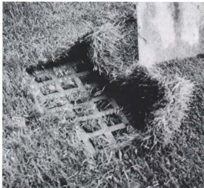
Turf growing through geomatrix grids buried below the surface provide extra protection against damage in high traffic areas.
