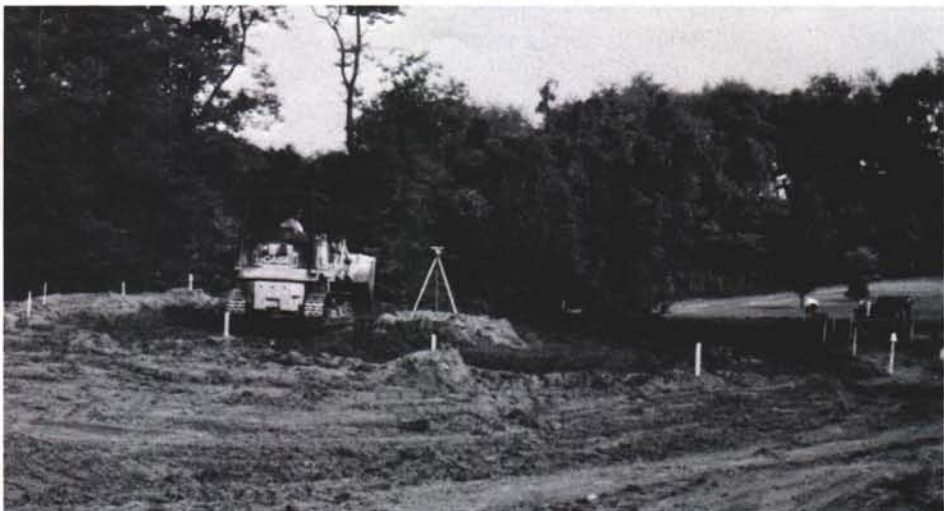
A dozer roughs out the perimeter of a relocated green to blend it into the "Scottish mounds" of the course.
