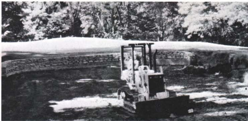
A lake was enlarged to increase the challenge of this rebuilt green. A field stone wall protects the edge of the green.
