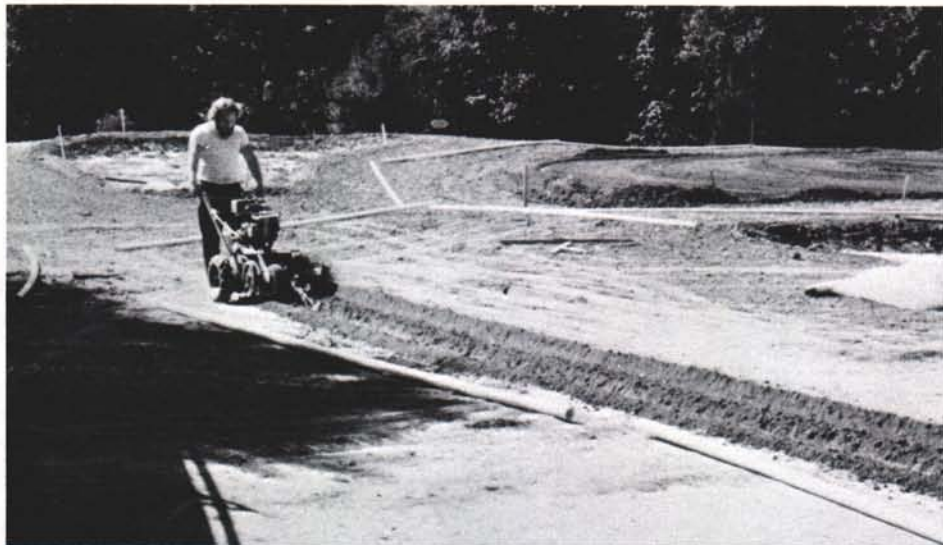
Miller and his crew install irrigation for a reconstructed green.
