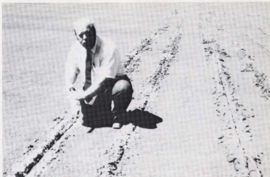
Dale Sandin examines the sand-filled slits cut into the field to restore drainage to the top six inches of amended sand on the PAT field.
