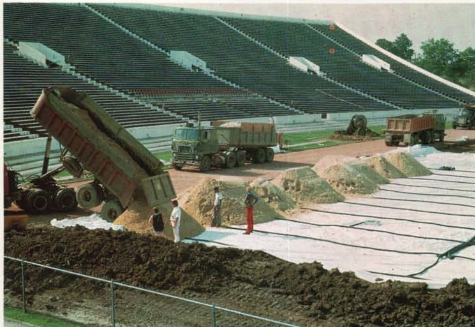
Fifteen inches of sand were spread over the plastic moisture barrier and network of perforated drainage pipe.
