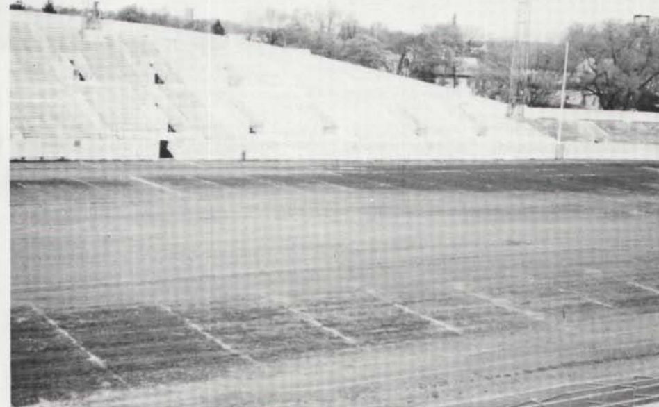
Worn-out football stadium field before renovation.
