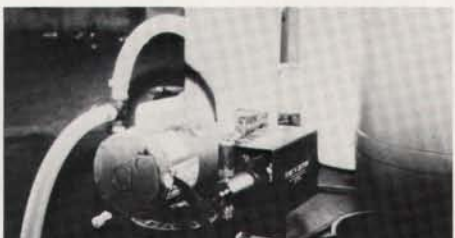
The injection pump was installed in less than a day providing Atlanta with new flexibility in fertilization.
