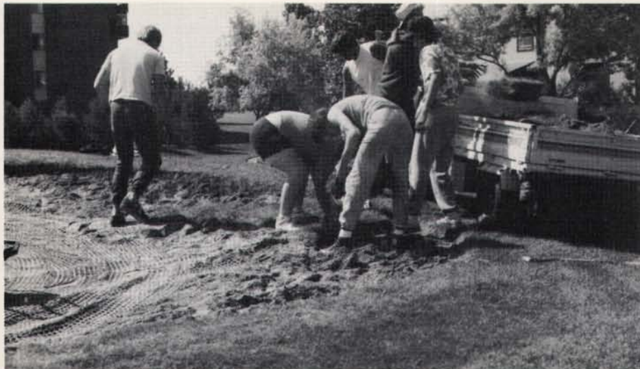
Auxer's crew restores a sand trap to its original shape and size. Turf had overgrown some traps by more than three feet.
