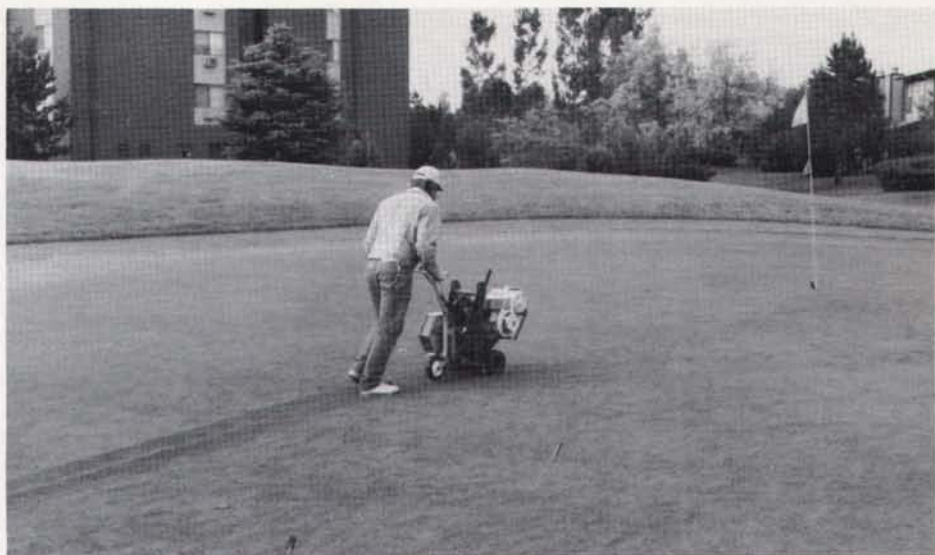
The installation process started by cutting a herringbone pattern in the bentgrass green with a sod cutter.
