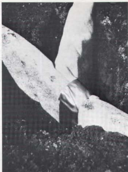
No special fittings are required to join together pieces of the drainage material, just duct tape.
