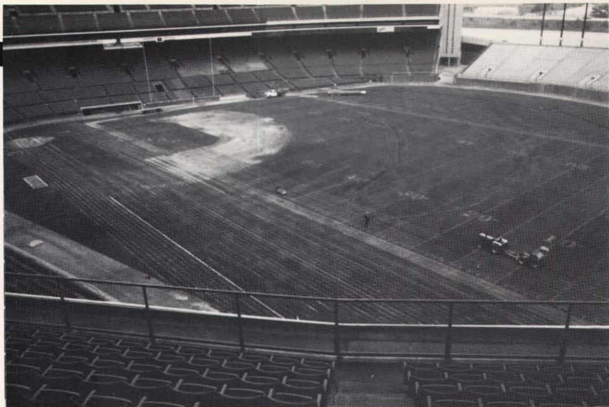
The narrow sand-filled trenches extended across the entire field. In less than a month, the new drainage system was hidden under spreading Kentucky bluegrass.
