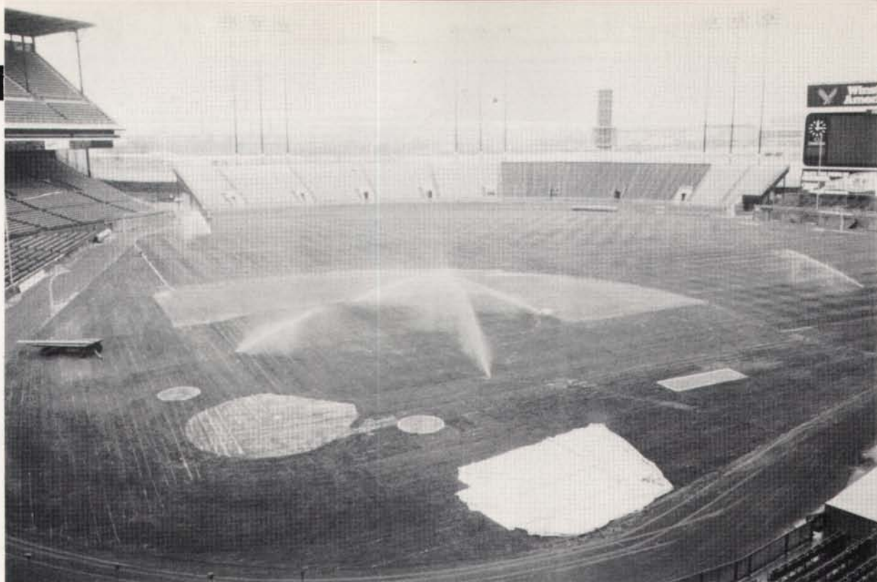
The first test of the infield irrigation was a success. The system lets Gill irrigate only the portions of the field that need water.
