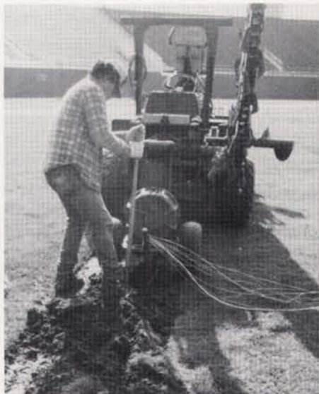
Pipes and wires were pulled into the outfield soil by a vibratory plow to keep disruption of the playing surface to a minimum.
