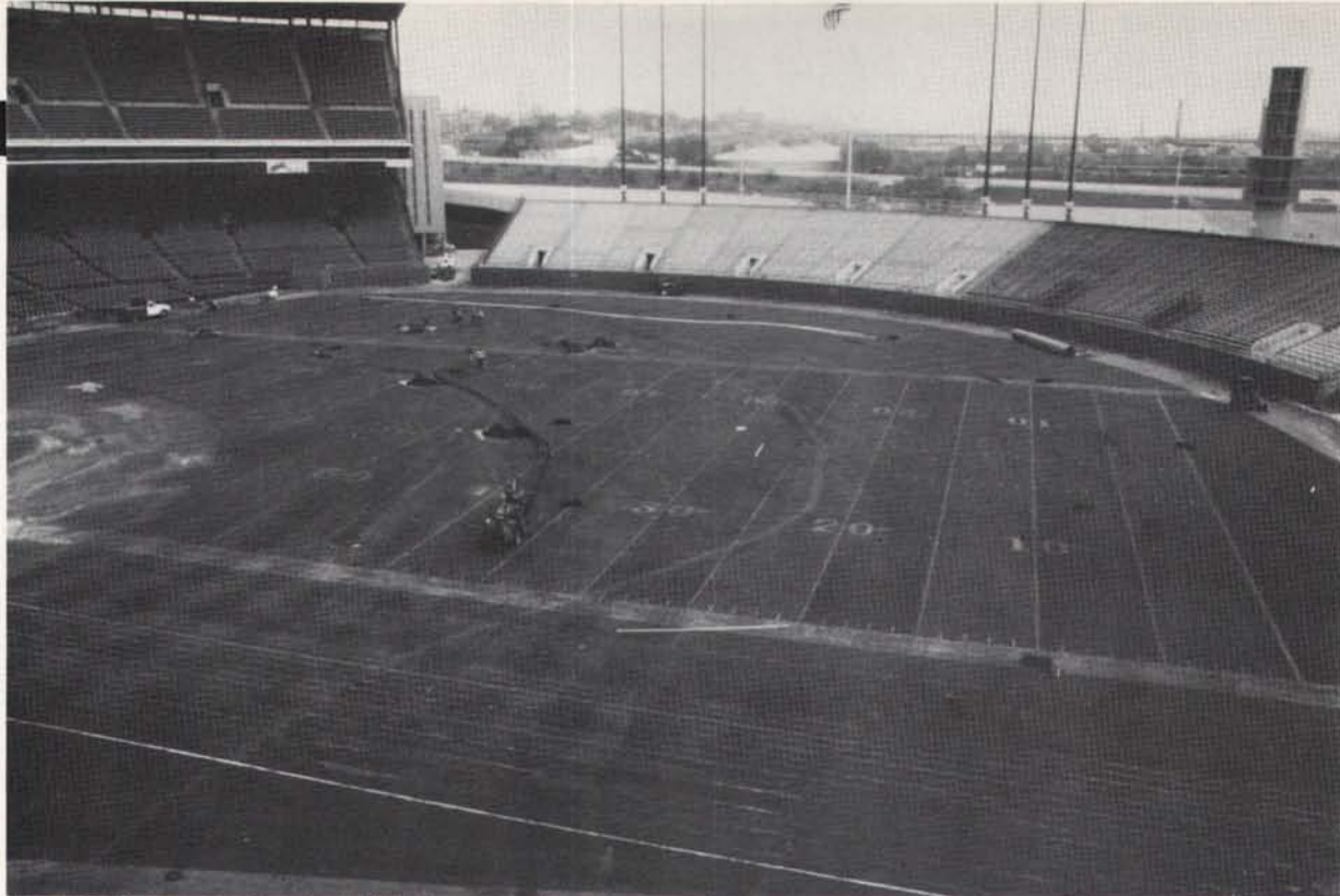
The irrigation contractors installed pipe and wires on one side of the field while the drainage contractor was sand-slitting on the other.
