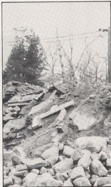
Debris removed from the top 12 inches of soil during reconstruction of a football field.
