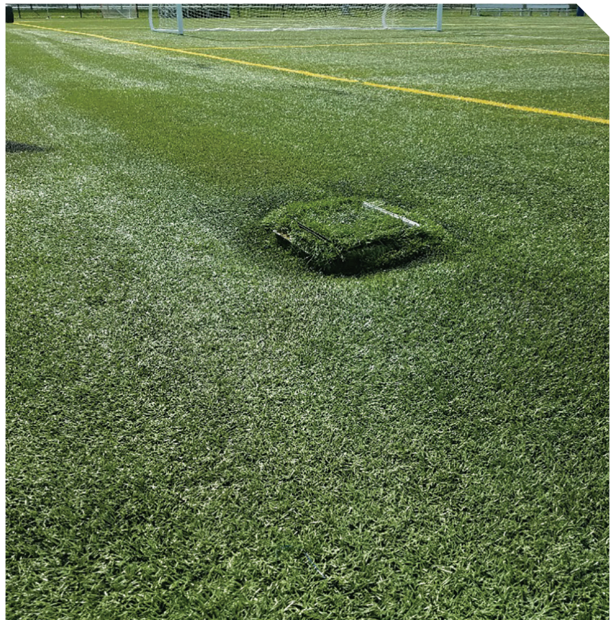
Sinkhole around a goal stabilizer.
