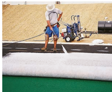
The type of spray rig that is frequently used to install these types of fields. Note that the 55-gal. drum is mounted on a portable carriage, along with the airless spray unit, so that the adhesive can be moved as the job progresses without any great effort. It also shows the adhesive being applied.
