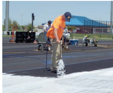
The first and perhaps the most important picture is the one showing the adhesive being sprayed with a spider-web pattern. Note also in the picture that the black sub-surface telegraphs through the white-sprayed adhesive indicating there are numerous places for the water to penetrate through.
