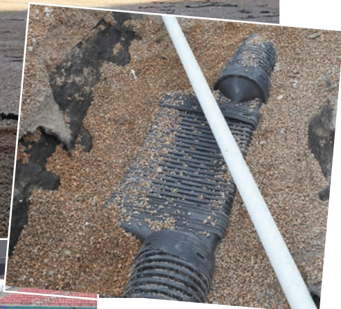
ADS Advantage piping was used for conflicts with irrigation.
