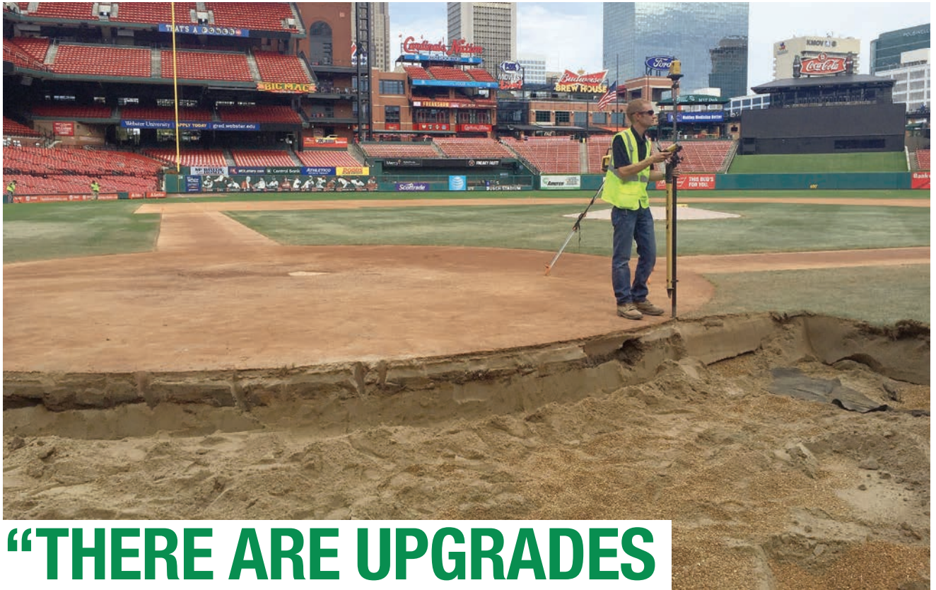
Derek York checking elevation.
