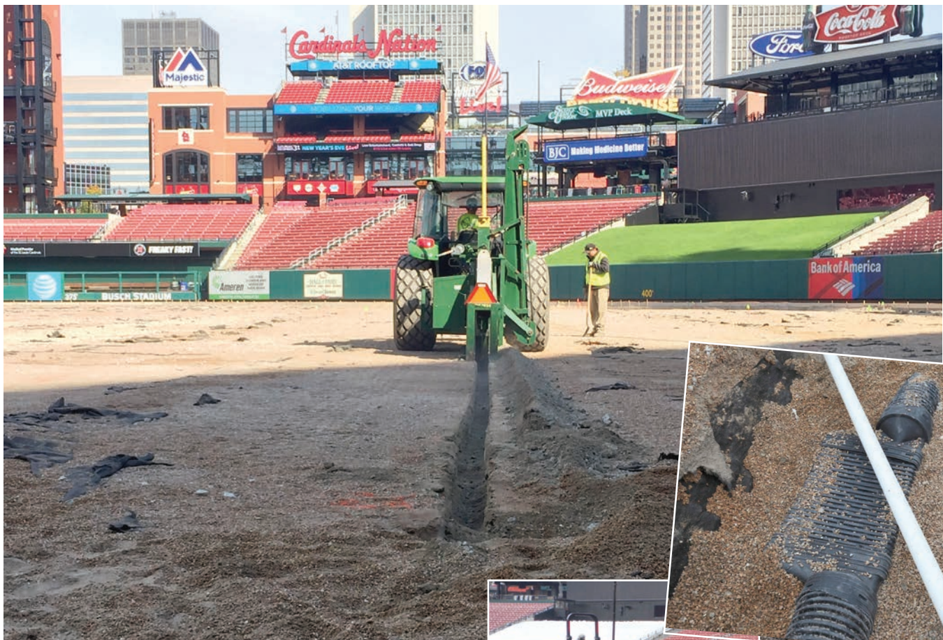
Trenching through concrete left over from old Busch Stadium.
