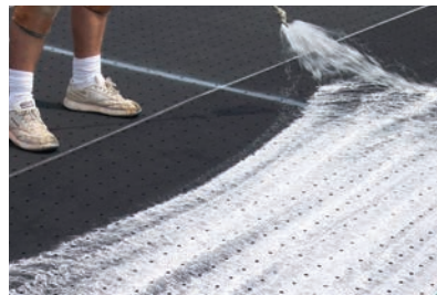
The second picture shows the adhesive being sprayed on a porous pad with holes drilled through for drainage. Note also, in the picture the spider-web pattern of the adhesive being sprayed.
