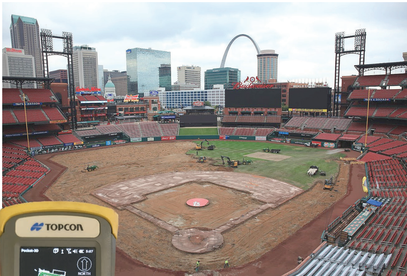
Removing the old field and grading base.
