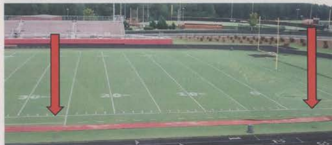
Figure 4. Locations of drains on the wrong side of a concrete runway causing water build up in the northeast corner of Field 2.
