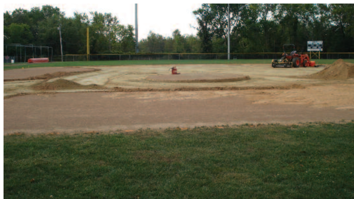
▲ After grading for surface runoff, 3 inches of skin soil is being removed in preparation for the new skin material.
