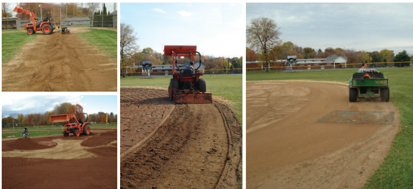
▲ Top Left: Excess skin soil is being removed from the base path to improve surface drainage. Bottom Left: A tractor is being used to spread the amendment evenly over the entire skinned area. Middle: The amendment is being rototilled into the existing skin soil at the recommended rate. Right: Notice the color is dull because the amendment is dusty from the tilling process.
