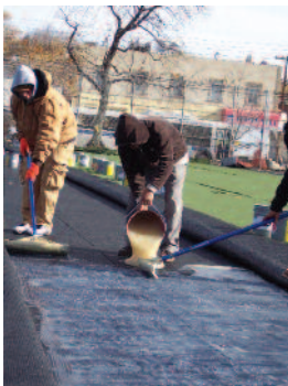
◀ Left: Airless Spray Center: Glue Box Right: Squeegee
