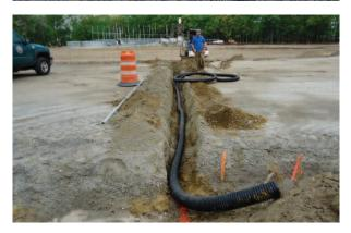
bottom of the trench slopes instead of the surface. This is particularly useful where there is limited area around the field. In addition, it is quite common to use a gravel trench drain to act as both a surface and subsurface drain.
