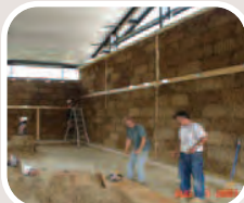
▶ Two of the walls here (one on the side and one on the back of the structure) are constructed out of bales of straw, covered in plaster. The highly compressed straw is fireproof and provides an outstanding level of insulation, using a renewable material.
