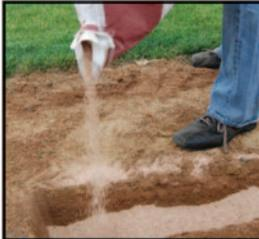
**Step 3:** For best results, slope the trench 1% from beginning to end. Ex: A 25 ft. long trench should have a pitch of at least 3 inches (25 ft. x .01 = .25 ft. or 3 in.).
