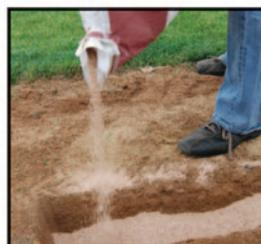
**Step 3:** For best results, slope the trench 1% from beginning to end. Ex: A 25 ft. long trench should have a pitch of at least 3 inches (25 ft. x .01 = .25 ft. or 3 in.).
