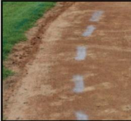
**Step 1:** Determine the length and number of trenches you will need. Every inch of depth in your trench, water will be pulled from 1 foot on either side of the trench.
