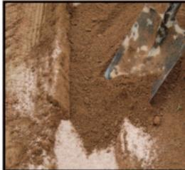
**Step 4:** Backfill all but the top inch of your trench(es) with Pro's Choice conditioner. Then add 1 inch of top soil to grade.
