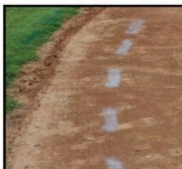
**Step 1:** Determine the length and number of trenches you will need. Every inch of depth in your trench, water will be pulled from 1 foot on either side of the trench.
