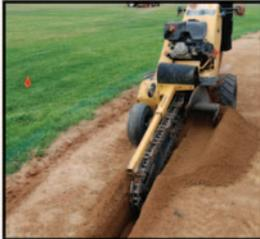
**Step 2:** Dig or use a walk-behind trencher. The size of your trench can vary. Many of the walk-behinds will cut a trench about 4 inches wide and 8 inches deep.
