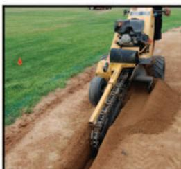
**Step 2:** Dig or use a walk-behind trencher. The size of your trench can vary. Many of the walk-behinds will cut a trench about 4 inches wide and 8 inches deep.
