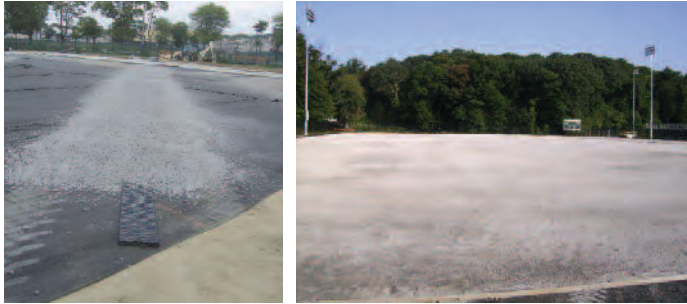
▲ LEFT: This cross-section shows the flat underdrain prior to installation in a field under construction. RIGHT: Sports field under construction showing the gravel drainage material.
