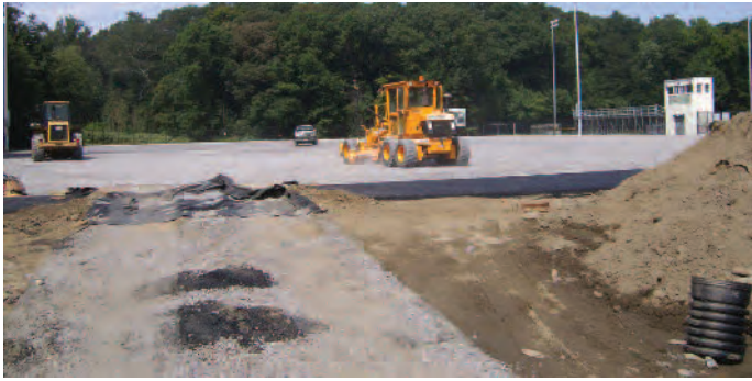
▲ A LAYER OF AGGREGATE is smoothed into place as part of the field construction process.
