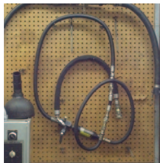
>> Bottom Left: THESE HOSES ARE FOR TESTING and draining a hydraulic system, which should be done at designated intervals, including during a winter service by a local distributor.
