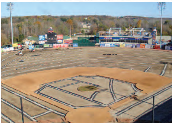
▲ Top: THE STRATEGY PLAN for the Lakes Community HS football field. Bottom: INSTALLED DRAINAGE at Fifth Third Stadium, home of the West Michigan Whitecaps.
