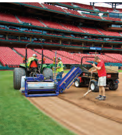
▲ Top: THE FINISHED PRODUCT. Photo by Taka Yanagimoto. Above Left: REMOVING THE INFIELD with a Terraplane rotor. Photo by Taka Yanagimoto. Above Right: REMOVING THE PITCHING MOUND. Photo by Taka Yanagimoto/St. Louis Cardinals.
