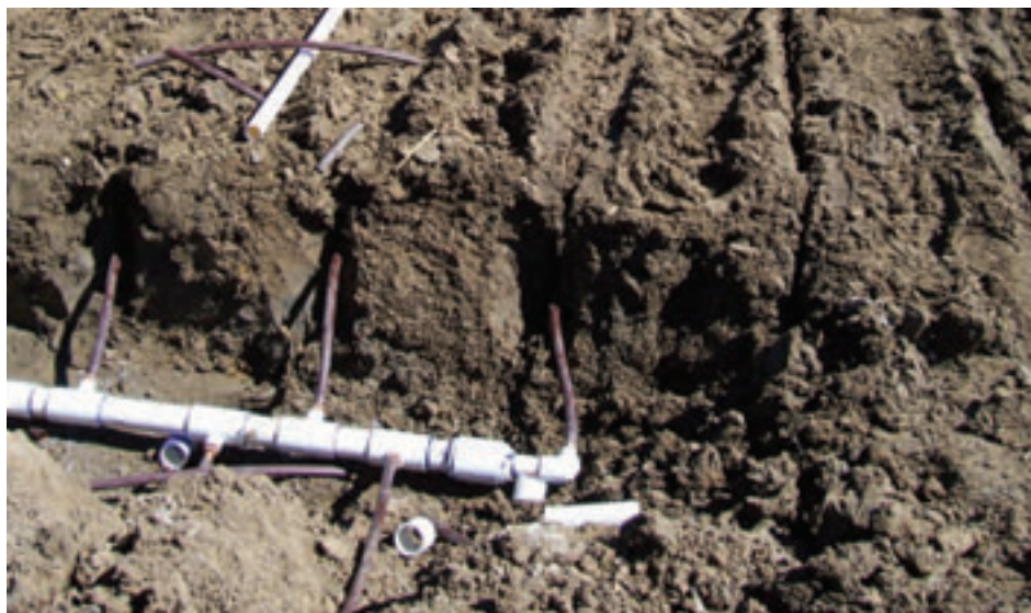
» NETAFIM TECHLINE CV DRIPLINE was run in lateral rows with approximately 14 inches between each line of tubing. The tubing was set in place with an automated Vermeer insertion plow.
